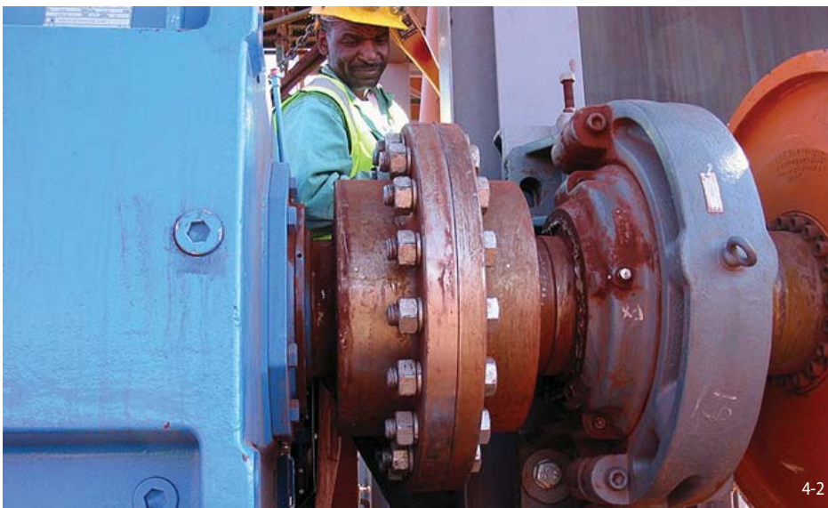
Tru-Line Flange-Coupling RFK 350 F - 350 M connects the gear of the drive unit to the head drum of an iron ore conveyor belt system in South Africa
